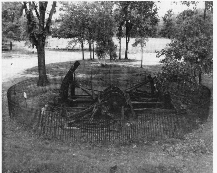
Waterbury's First Brass Mill Wheel Demolished By Storm
